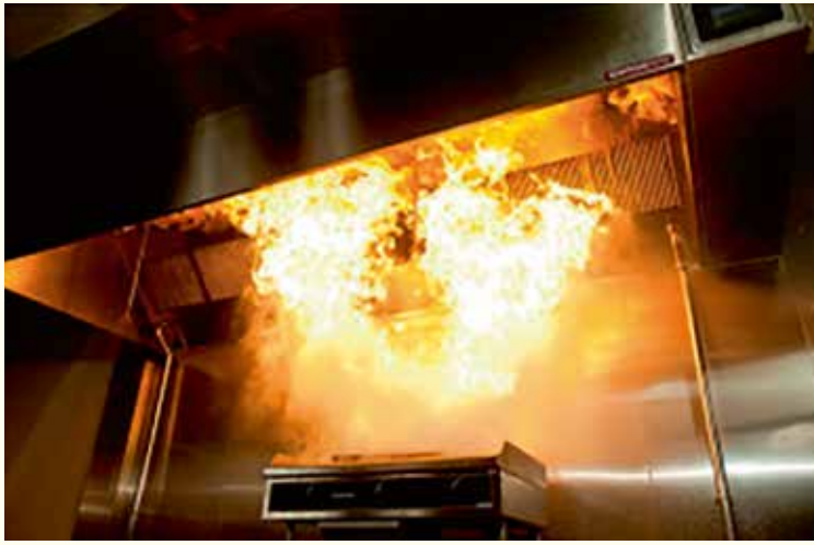
A fire within the duct can ignite combustible materials outside of the duct, spreading the fire in the building.
